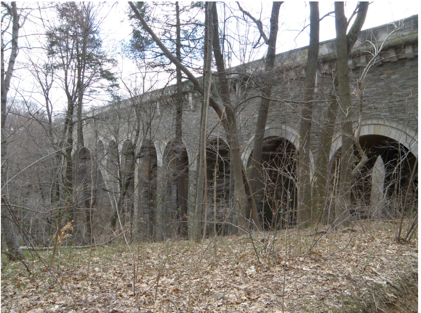
Stone Faced Concrete Arch Bridge
